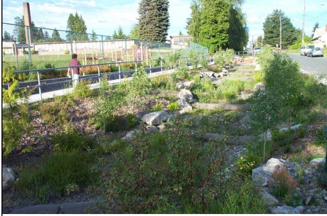
Image 6-10. Vegetated Swale, Maria Cahill. Water-quality swales: Low-impact development fact sheet. (2018, June 1). OSU Extension Catalog, Oregon State University. Retrieved October 7, 2021, from https://catalog.extension.oregonstate.edu/em9209/html .
