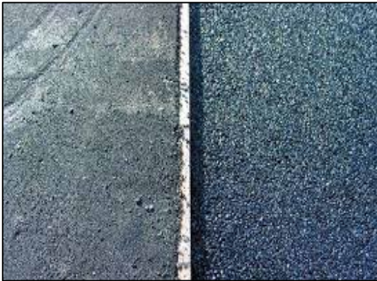
Porous Asphalt. Source: Cornell University Urban Horticulture Institute. (2007). Using Porous Asphalt and CU-Structural Soil®. Retrieved October 7, 2021, from http://www.hort.cornell.edu/uhi/outreach/pdfs/cu_porous_asphalt.pdf .
