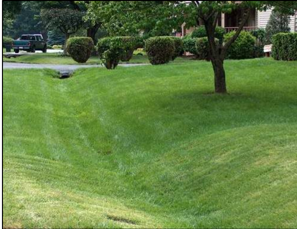
Grassy channel. Source: Fairfax County Virginia. (n.d.). Control Heavy Runoff - Solving Drainage and Erosion Problems. Retrieved October 6, 2021, from https://www.fairfaxcounty.gov/soil-water-conservation/drainage-problem-control-runoff .
