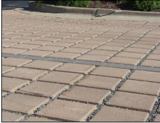
Pervious Pavers. Source: Bay, A. for the C. (n.d.). Reduce your stormwater. Pervious Pavers. Retrieved October 7, 2021, from https://www.stormwater.allianceforthebay.org/take-action/installations/pervious-pavers .
