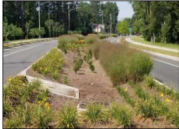
Roadway Bioretention Areas in Raleigh, NC. Source: Raleighnc.gov. (n.d.). Retrieved October 6, 2021, from https://raleighnc.gov/SupportPages/roadway-Bioretention-areas .
