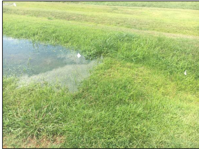
Grassy Swale. Source: Ekka, S., & Hunt, B. (n.d.). Swale terminology for urban stormwater treatment: NC state extension publications. Swale Terminology for Urban Stormwater Treatment, NC State Extension Publications. Retrieved October 7, 2021, from https://content.ces.ncsu.edu/swale-terminology-for-urban-stormwater-treatment .
