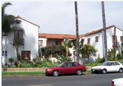
Building B Density: 31.7 du/ac. Number of units: 8 Building footprint 84'x32' (rear bar), 31'x25' (side bars)', 2 Stories
