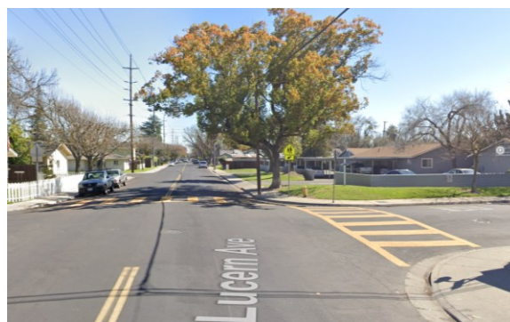
Figure 4: Crosswalk Striping (Lucern Ave)
