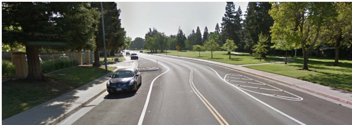
Figure 14: Striped Chicane
