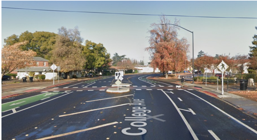
Figure 13: Median with Pedestrian Refuge (College Avenue)
