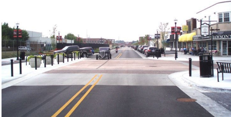
Figure 9: Raised Intersections
