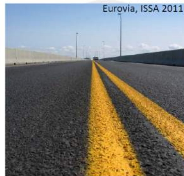
Confederation Bridge, Canada
