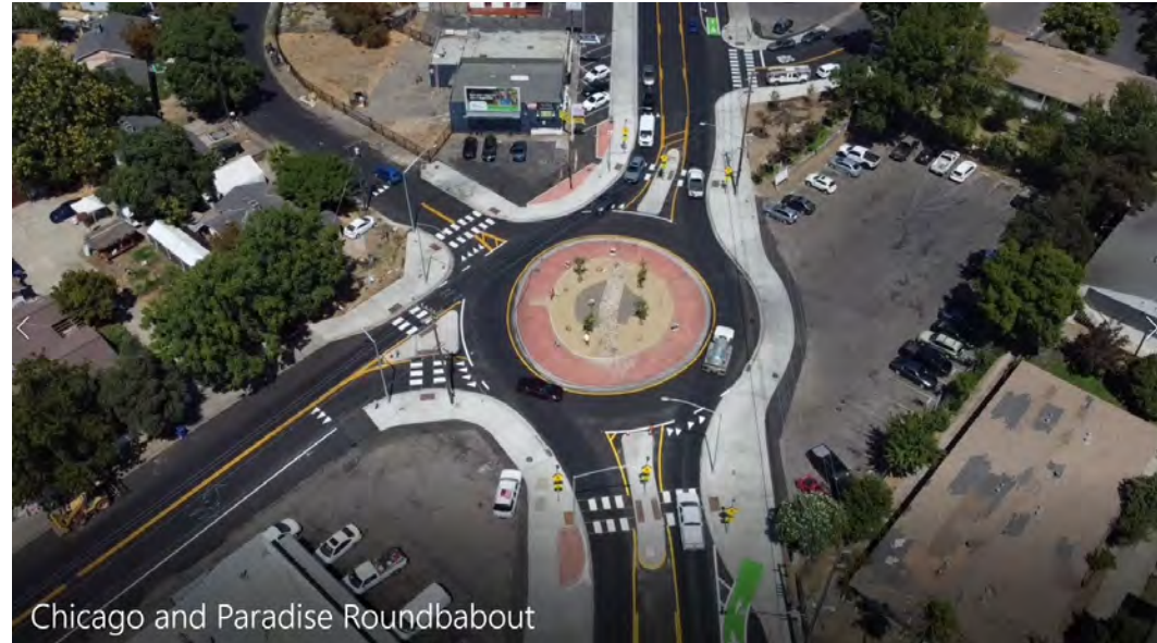
Recently Constructed Paradise and Chicago Roundabout
