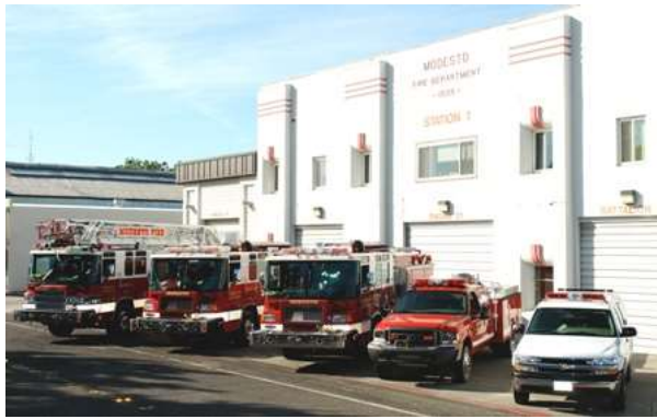
Figure 94 : Modesto Fire Department Station 1
