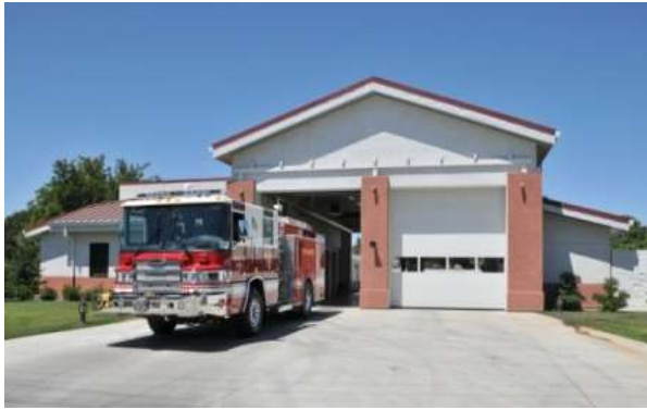
Figure 95 : Modesto Fire Department Station 2
