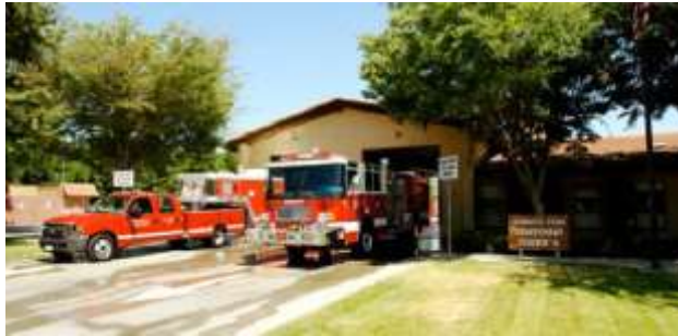
Figure 97 : Modesto Fire Department Station 4
