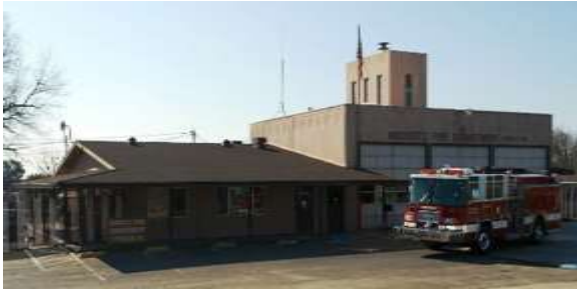
Figure 103 : Modesto Fire Department Station 10
