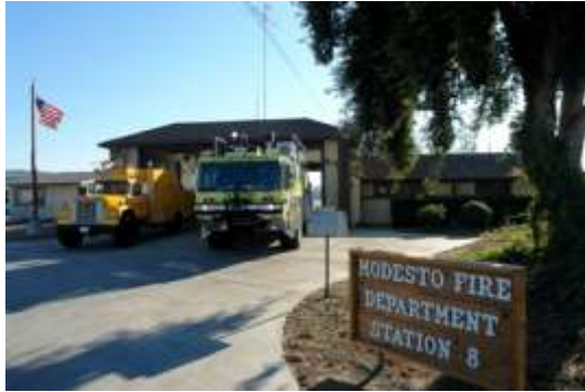
Figure 101 : Modesto Fire Department Station 8
