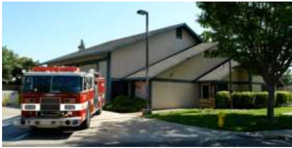
Figure 102 : Modesto Fire Department Station 9
