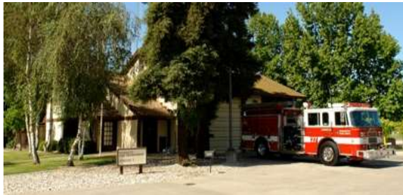
Figure 100 : Modesto Fire Department Station 7
