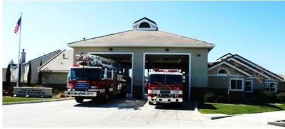
Figure 104 : Modesto Fire Department Station 11
