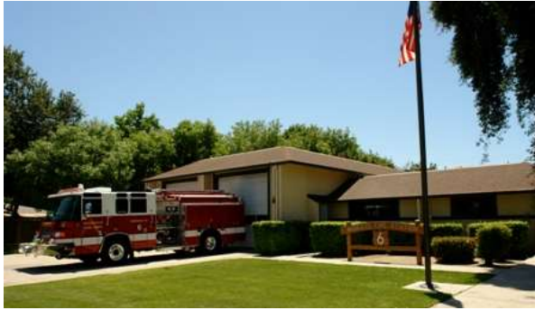
Figure 99 : Modesto Fire Department Station 6
