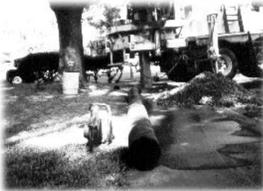
pressure on the core pipe is so strong that it unravels and looks like a cork screw. When it is finally out they attach a huge bucket-like drill bit to a long pole. The long pole pushes down into the drain and bores deeper. It continues drilling until it reaches its maximum depth. This process is about 97 percent successful.
